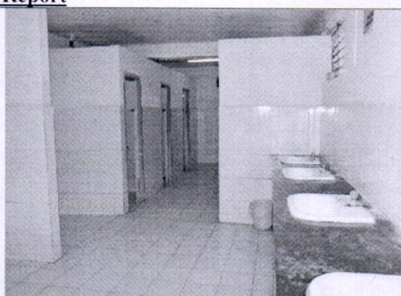
Improvising the basin cabinet in the Boys Hostel
