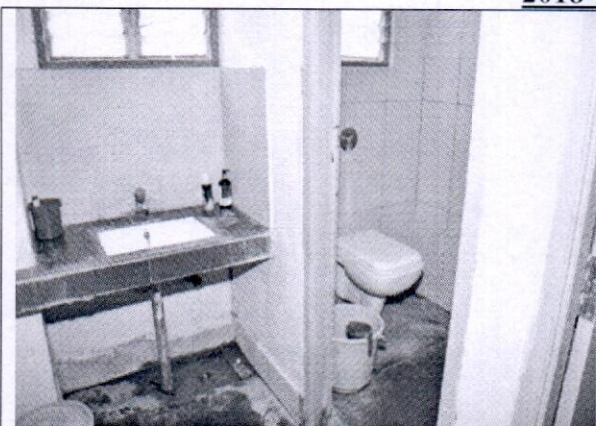
Improved toilet facility in the VFSTR
