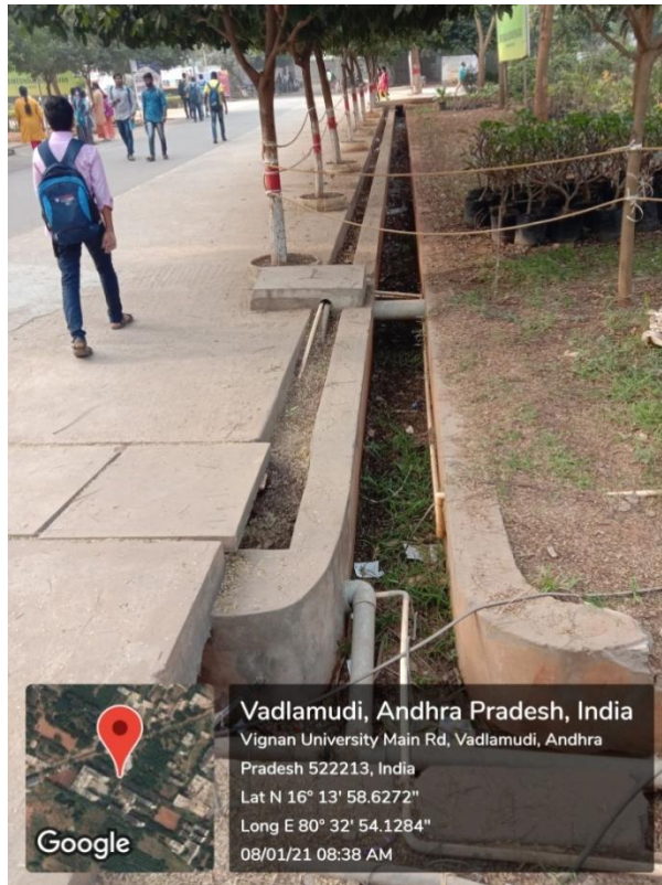
Fig 17. Open Drains at VFSTR campus
