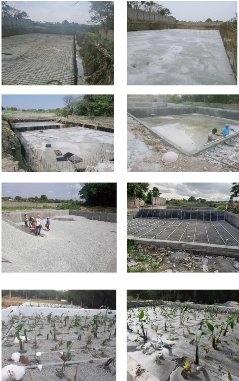
Fig 15 Execution of STP at VFSTR-Constructed Wetland
