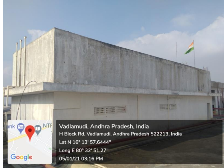
Fig 11. 38,500 Litres capacity tank at H-Block, VFSTR
