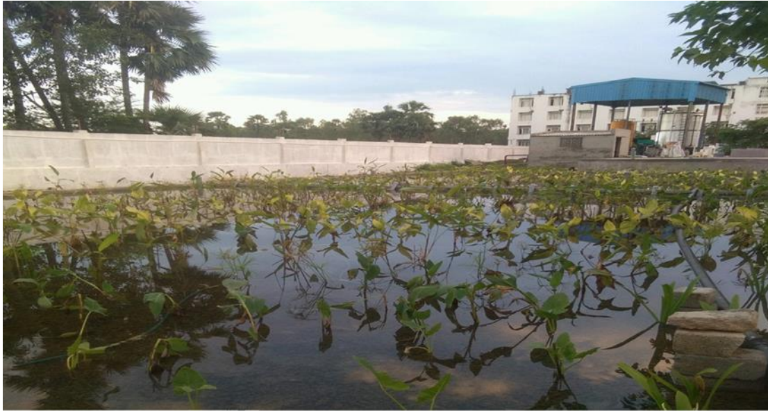
Figure 5: Sewage Treatment Plant at VFSTR
