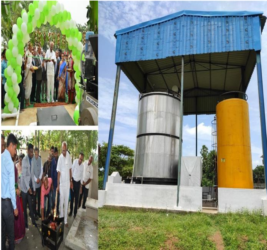
Figure 2: Biogas Plant at VFSTR campus
