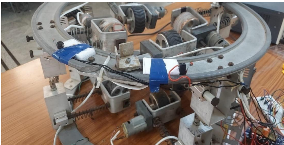
Fig 2.2: Installation of Limit switches
