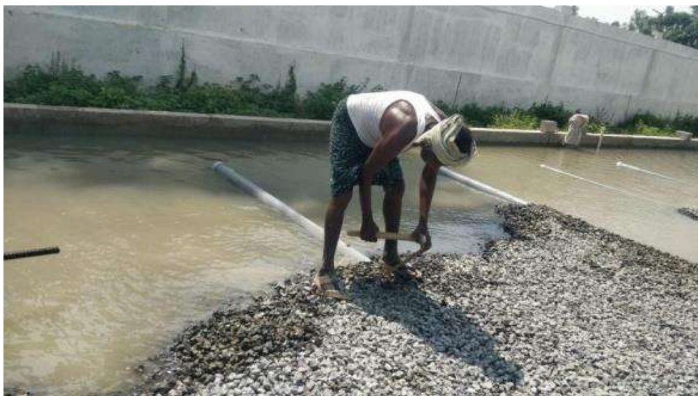
Local gravel (20mm size) – 1500 Tons of local 20mm Gravel has been used
