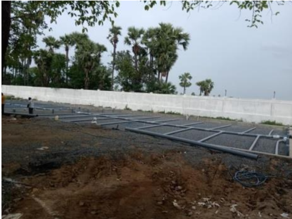
Treated Network @ 1.8m from RCC Raft
