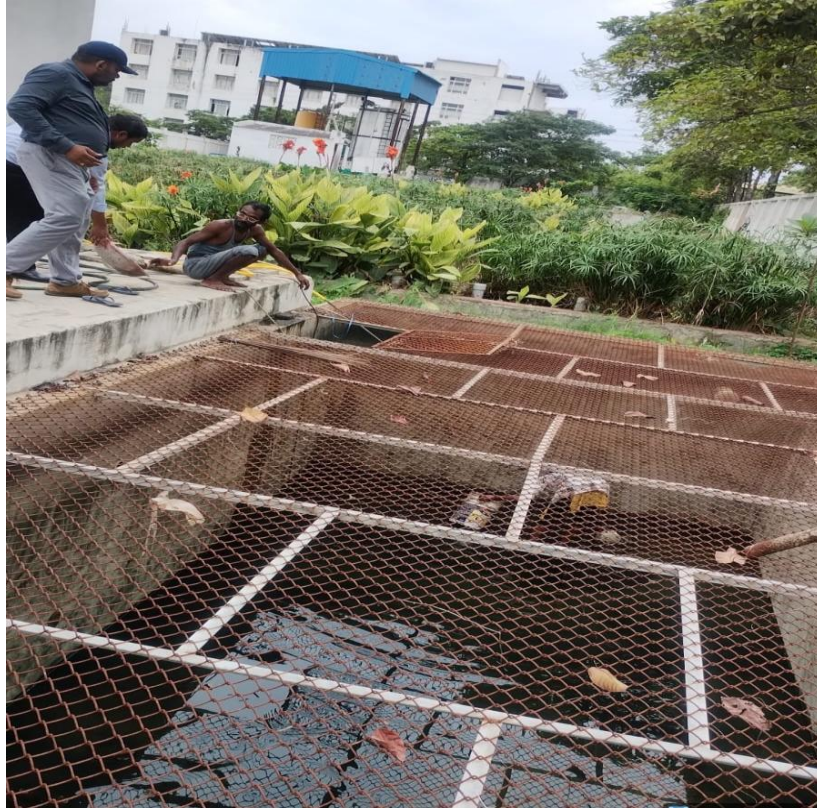
Clearance of Grit and removal of settled sludge in Tertiary Tank
