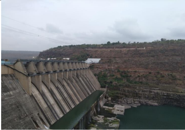
Fig.18: Side view of Srisaillam dam
